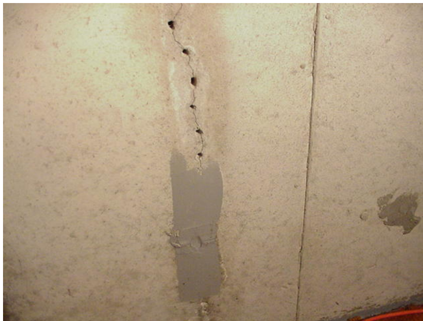
Figure 8-4 Use of Sealants to prevent Vapor Intrusion Through Cracks
