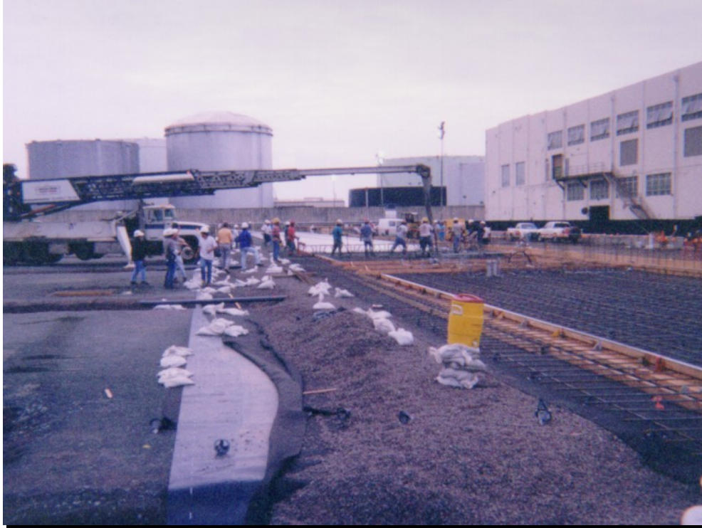
Figure 8-5 Multiple Layers for Venting Being Installed Prior to Construction
