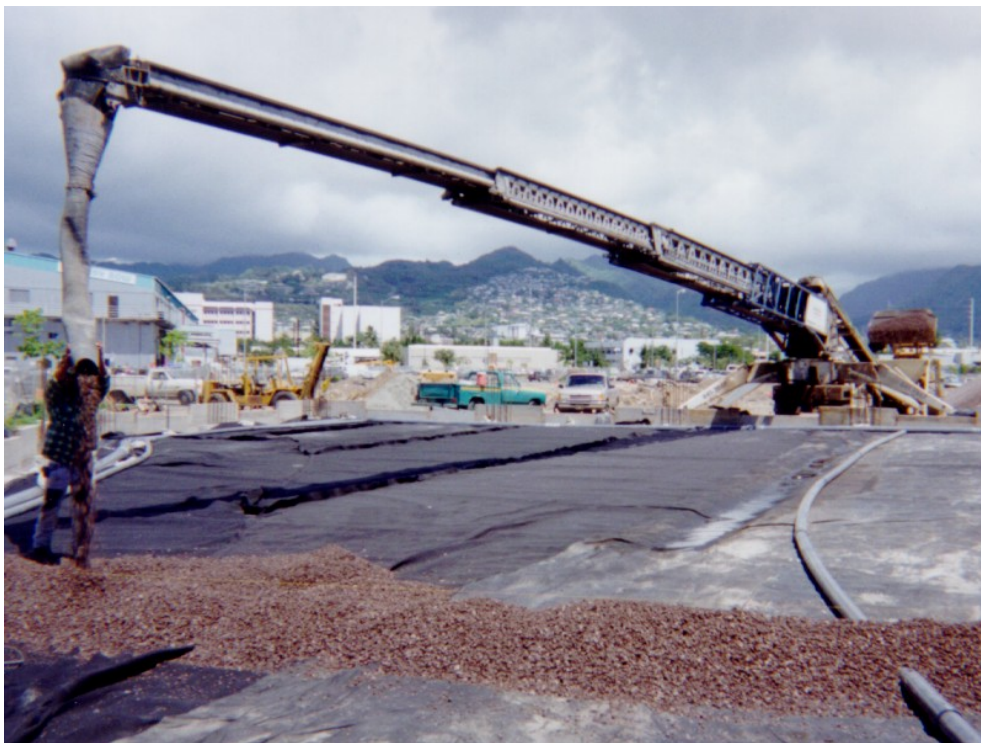
Figure 8-5 Multiple Layers for Venting Being Installed Prior to Construction
